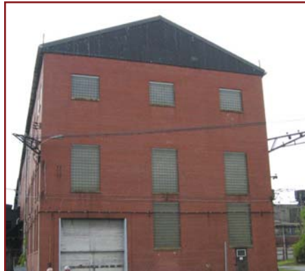
120" Rolling Mill Motor House exterior, looking west
