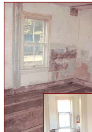
Tenant House interior before and after restoration
